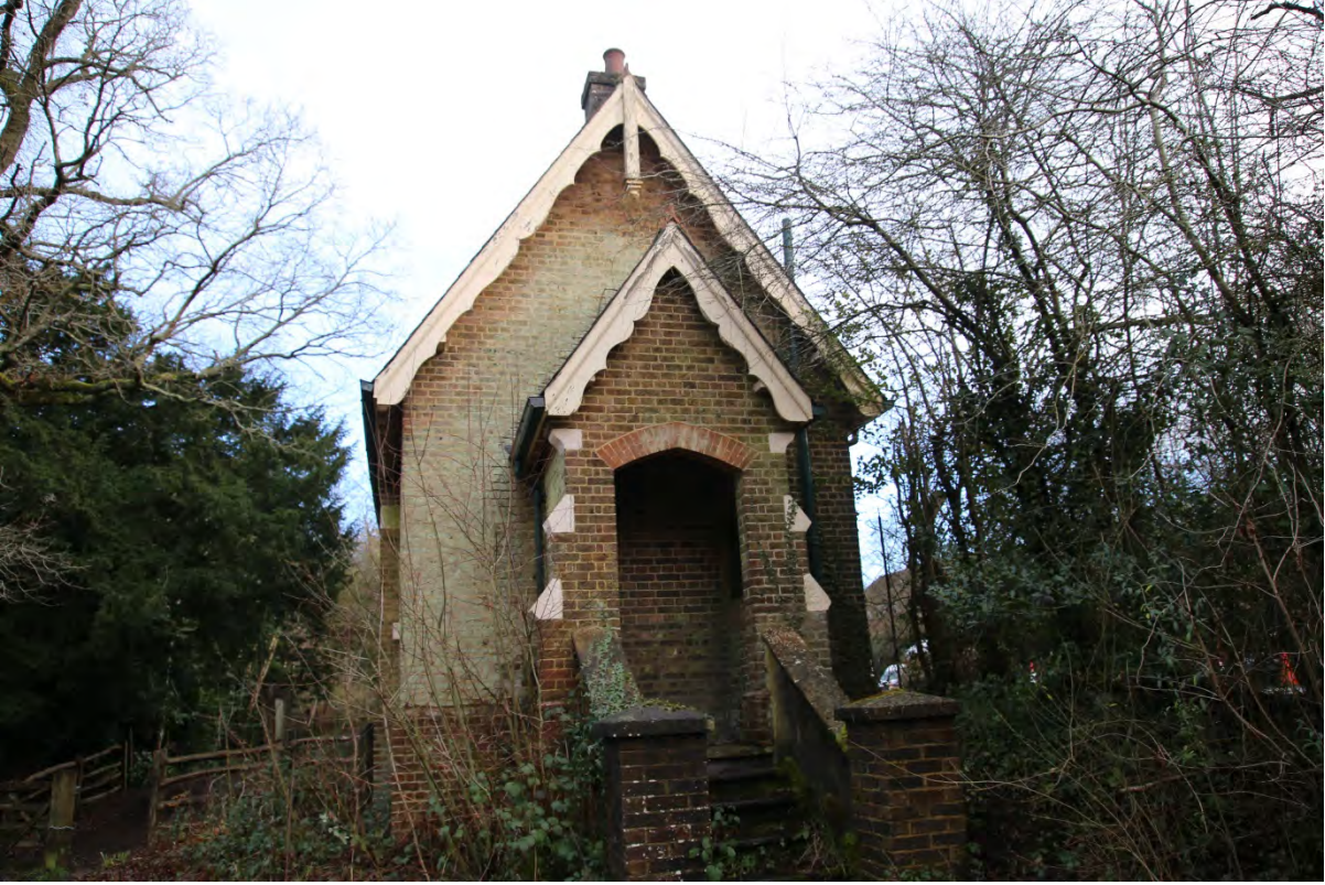
Rowfant Estate shelter at Railway Station
