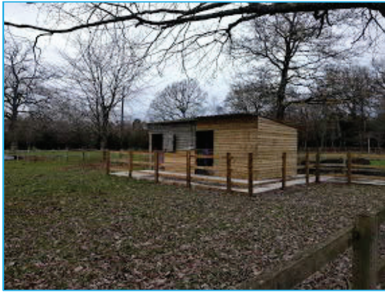
Photo 1 Stable building (B1)-negligible suitability for roosting bats
